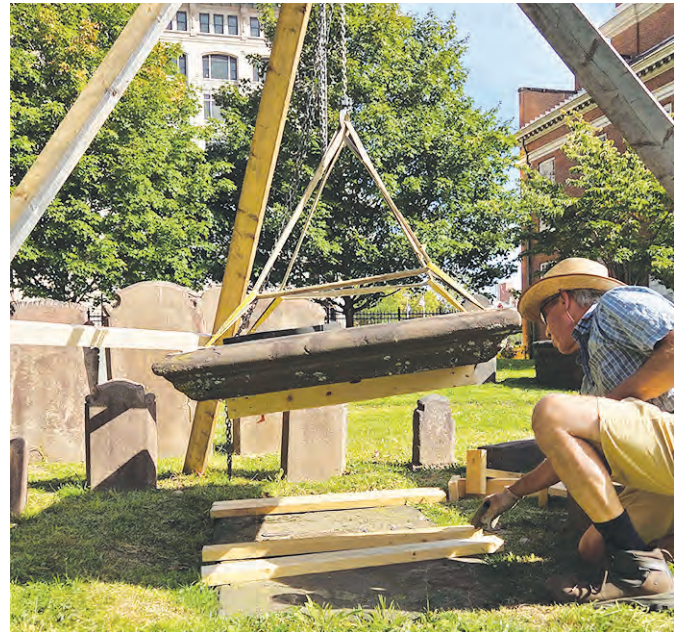
Jonathan Appell of Atlas Preservation dismantled the 1500 lb. tablestone of John Ellery without mechanical equipment or extra help. Jonathan was able to skillfully "walk" the massive stone away from the base, leaving the base and legs accessible for conservation work.
